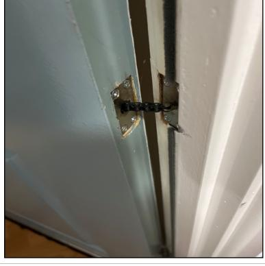
Door is fitted with a concealed self-closer (perko) closer and does not fully self-close
