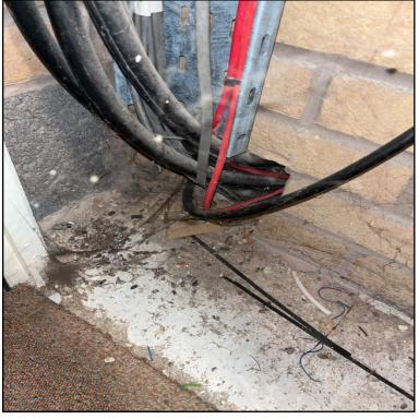
Services penetrate the compartment wall without adequate fire stopping
